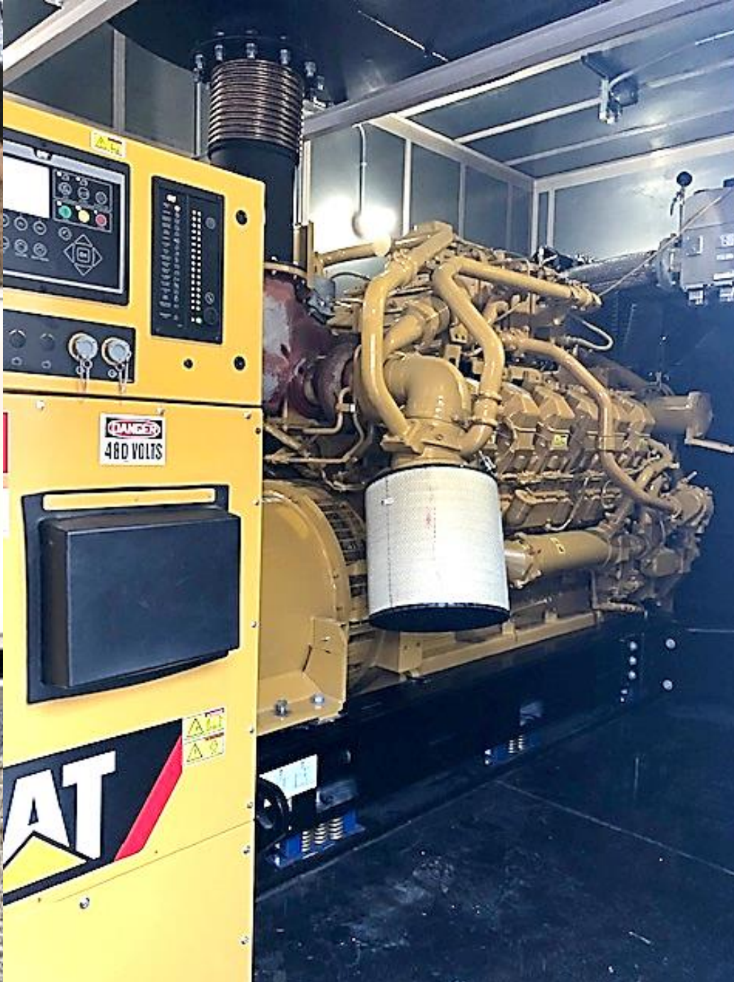
Natural Gas Powered Back-up Generator
